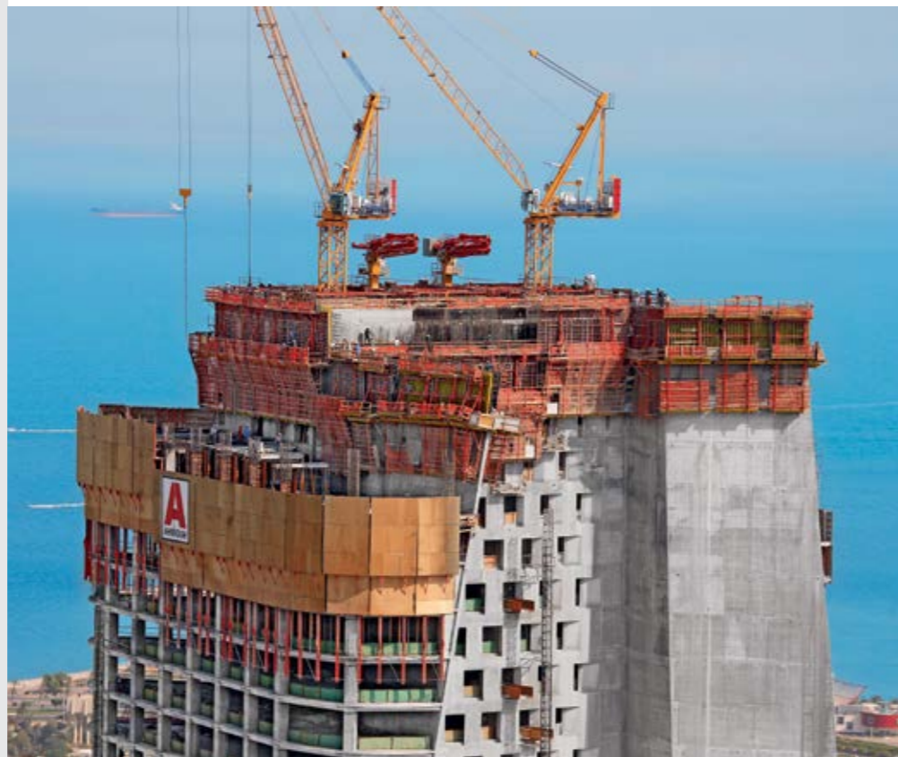
Picture source: PERI GmbH, Weissenhorn
